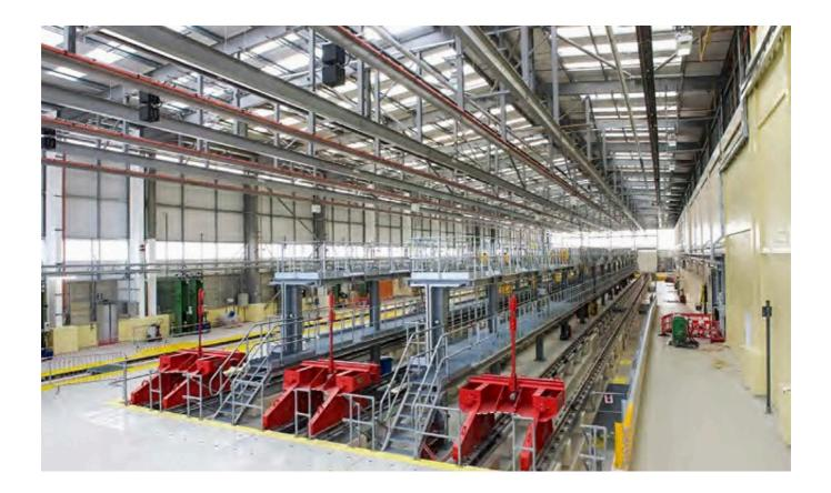
The project included the improvements and conversion of New Cross Gate depot from a 4-car to a 5-car facility for London Overground. The project included extension and modifications to the main maintenance building, wheel lathe Building (including new wheel lathe pits), relocation and extension of the 25kV test track and reconfiguration of the stabling roads within the Depot to accommodate 5-car trains.
