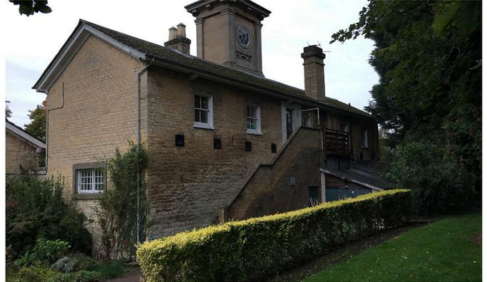
The building comprises traditional construction with Ashlar stone facework secured to the inner stonework with iron or wrought iron clamps. The roof is a mixture of pitched and flat roofs with slate and lead roof coverings, supported on a timber rafter and purlin roof structure. A feature timber roof light called the East Lantern was in place which allowed natural light into a two-storey atrium and stair area.
